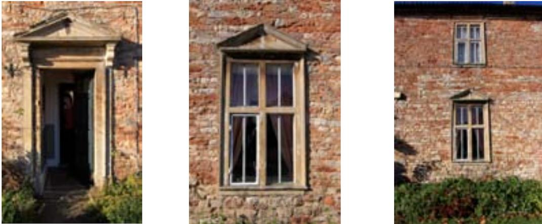
The classical detailing of the door and window openings within the facade
