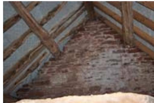
Contrasting replacement and historic timbers in evidence in the roofing pattern
