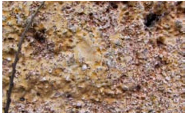
Red sandstone 'brickwork' polite finish in contrast to the harling render and limewash finish of the rear elevation
